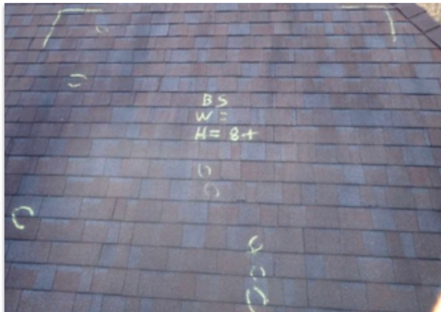
Photo 2: Back slope test square overview
