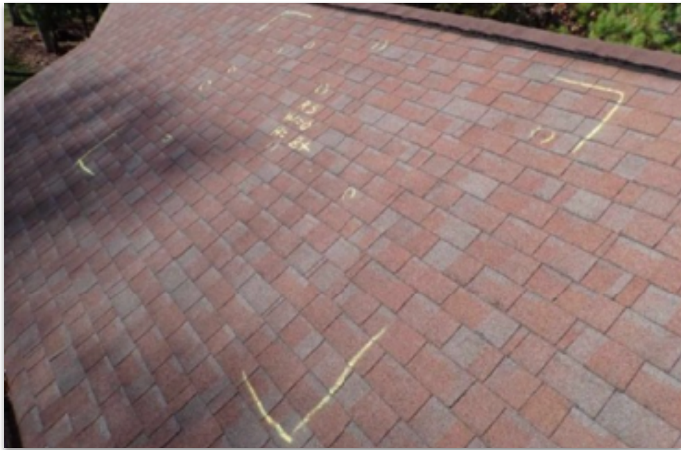
Photo 3: Right slope test square overview
